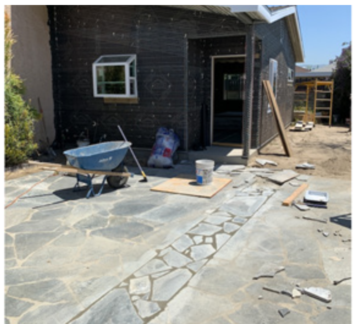
Examples of backyard excavations for sewer, water, and electricity
